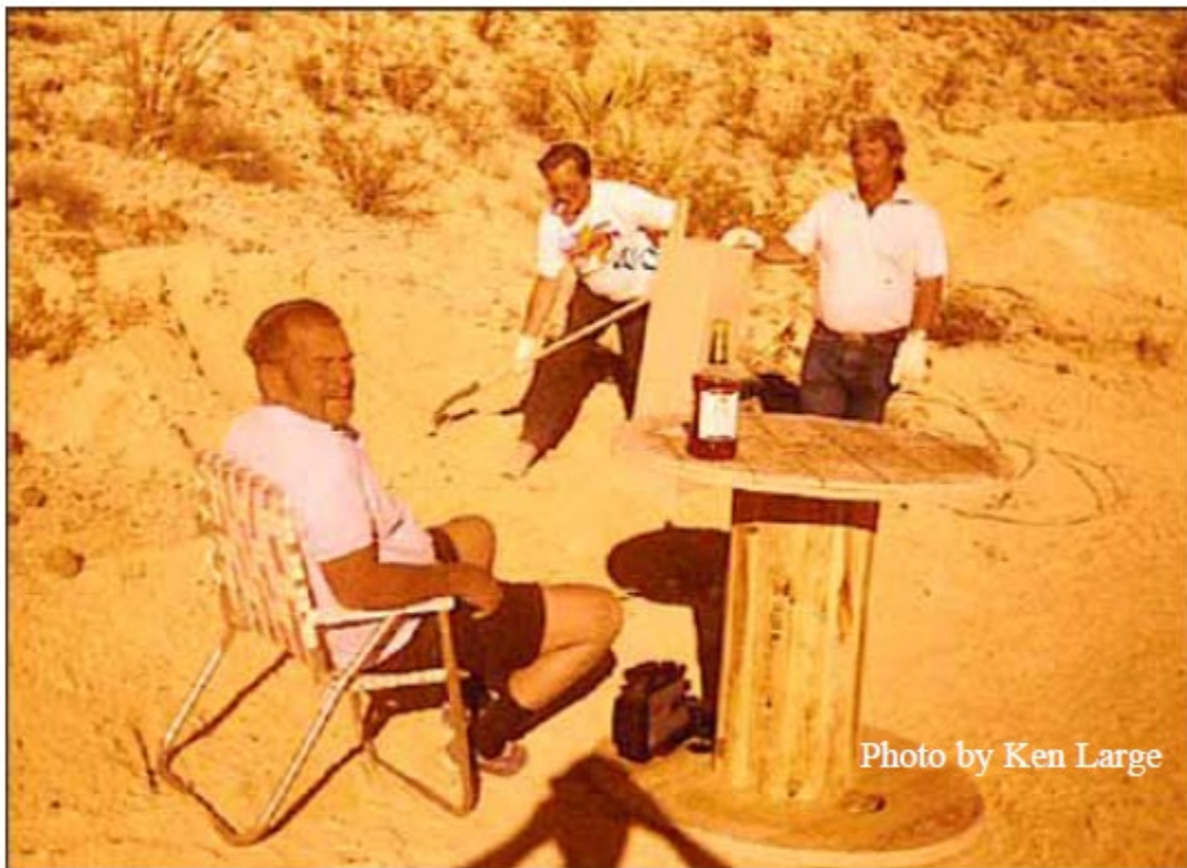
A weedy row, a dull hoe and a mean boss. Bill Simpson, Ed Kelley and Jerry King putting the finishing touches on cable installation.
